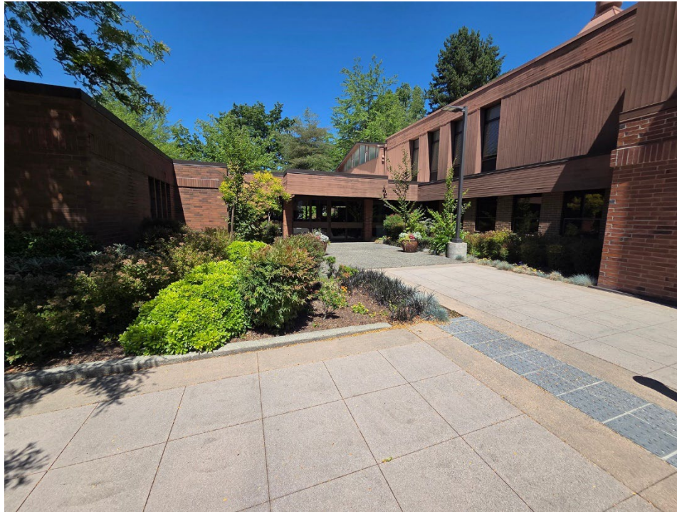
Plate 1. Proposed addition location, looking north (7/8/2025).
